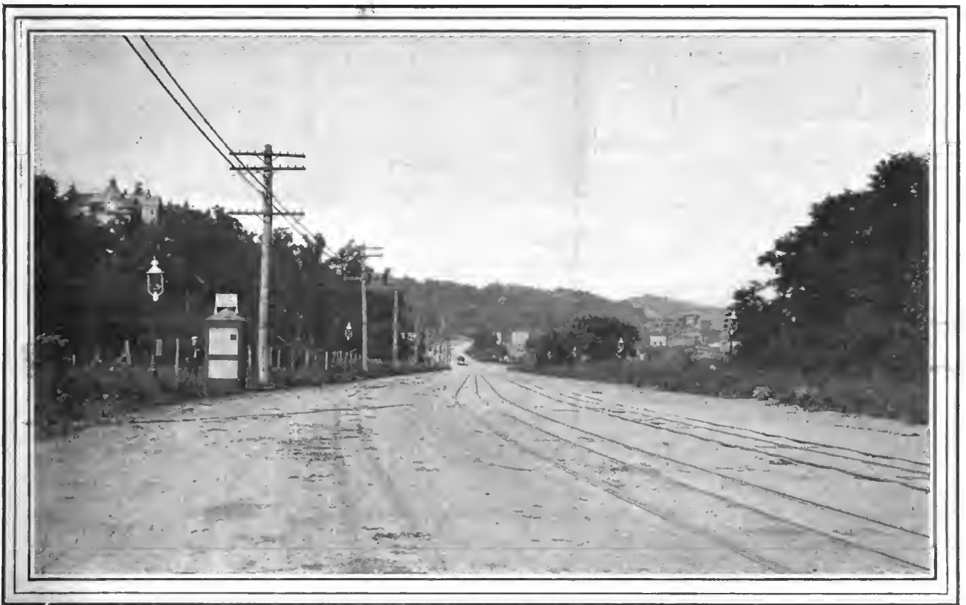
KINGSBRIDGE ROAD, NEW YORK CITY, LOOKING NORTH FROM 190th STREET, SHOWING NEW POLICE SIGNAL BOOTH ON WEST SIDE. Second Station Is Located at Foot of Grade, Near Trolley Car, and Third Is Near Last Turn of Road in View.
